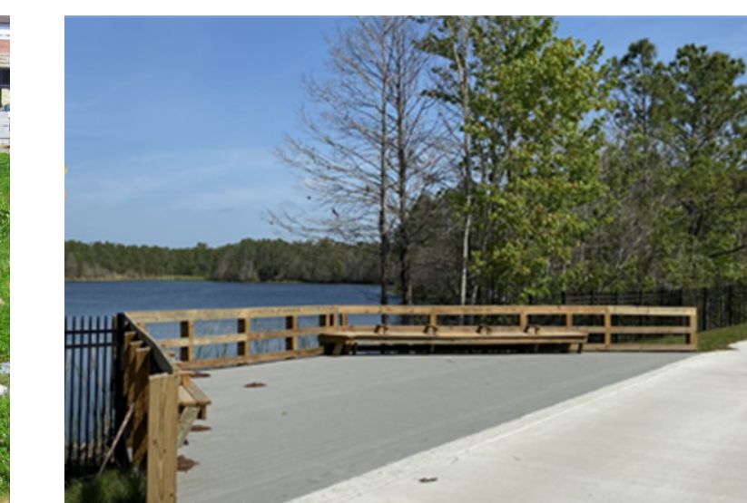
Stream Overlook Single Creek Trail Overlook, Florida
