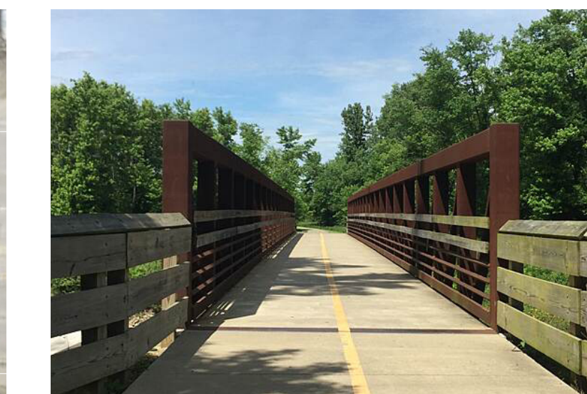
Pedestrian Stream Crossing Armler-Lurken Connector Trail Duck Creek Bridge, Ohio
